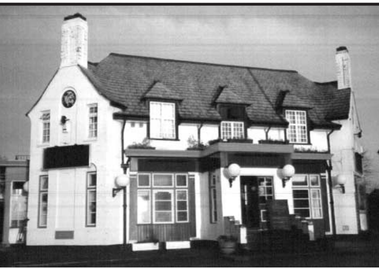
A fond farewell...to The Manor Cottage, East End Road. Recently demolished to build a selection of two-bedroom flats. Photo by Alison Roberts
