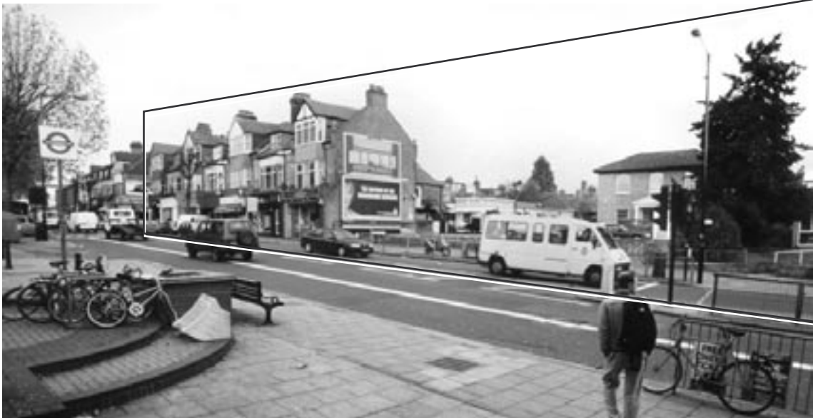
The site of the proposed Waitrose and library development - photo by Erini Rodis. We have marked the extent of the development on the photo above, which is taken from outside the railway station. To the right the development stretches out of site, almost to Cherry Tree Wood. The shops as far as Baronsmere Road are included.
