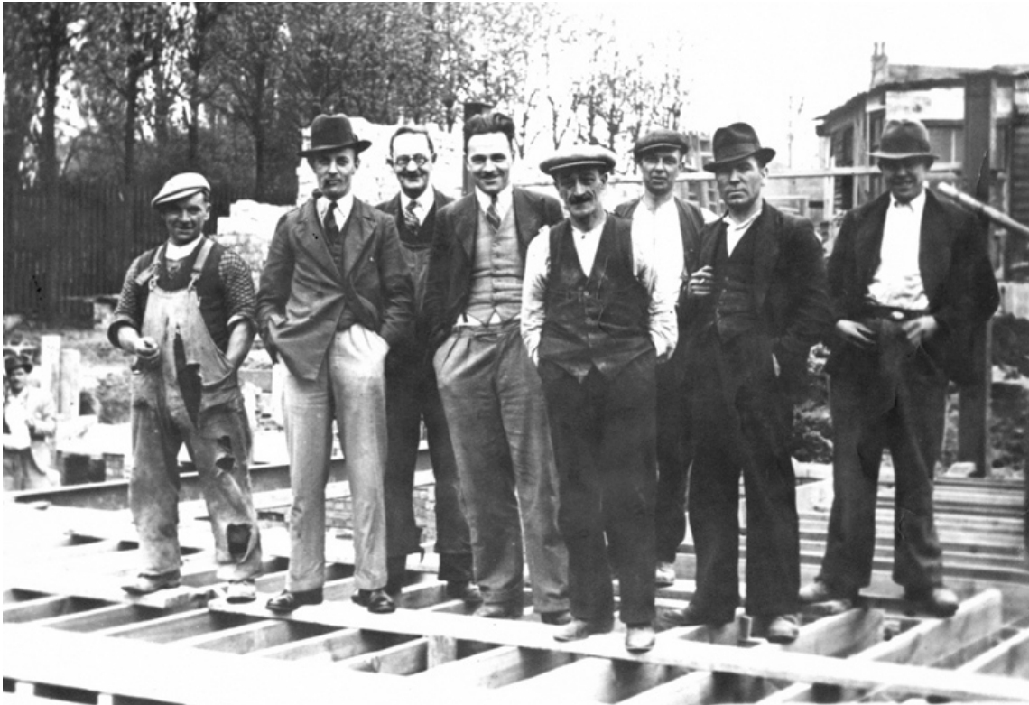
Builders of the Northern Line. Photo supplied by Audrey Cartwright.
