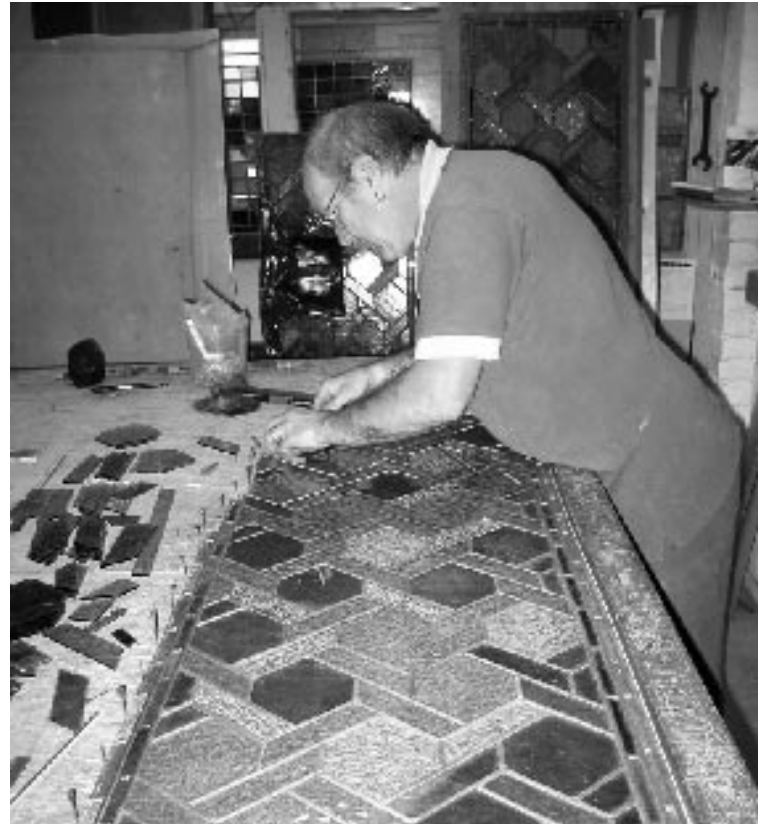
A craftsman at Gilbert and McCarty (stained glass restorers) working on one of the three damaged windows at All Saints Church (see letter below). This firm put back the glass on Big Ben when it was last reconditioned and did restoration work at Windsor Castle after the 1992 fire. Photo: M. Bronkhorst
