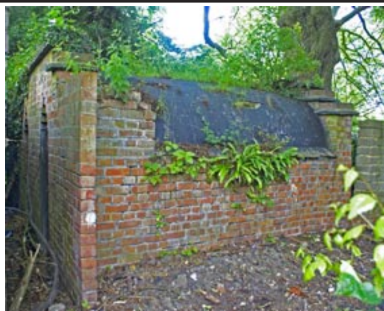
The air raid shelter in East End Road. Photo by Craig Johnson
