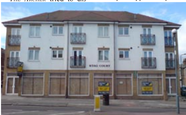
The ground floor of Stag Court is still vacant. Photo by John Lawrence
