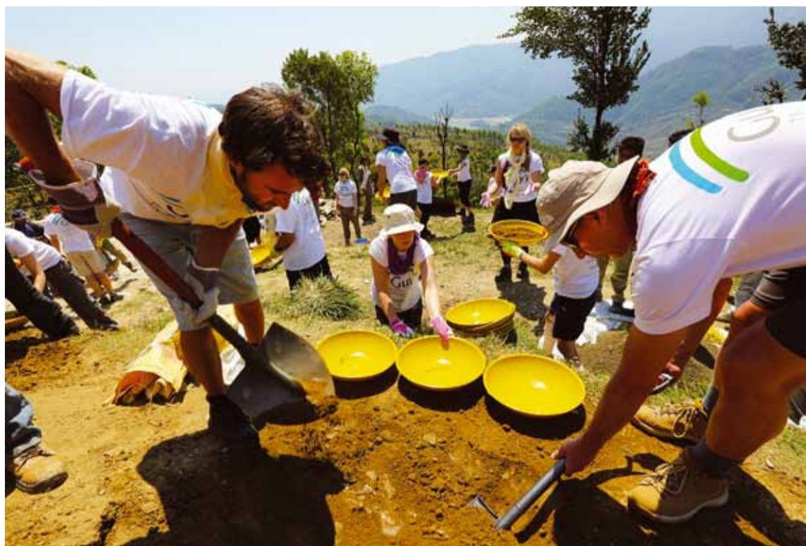
The Guy's Trust team start digging for the new village school
