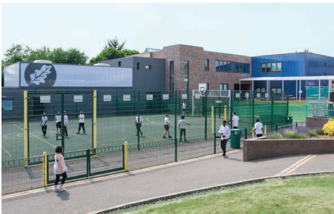
The new block at Oak Lodge School. Photo Mike Coles
