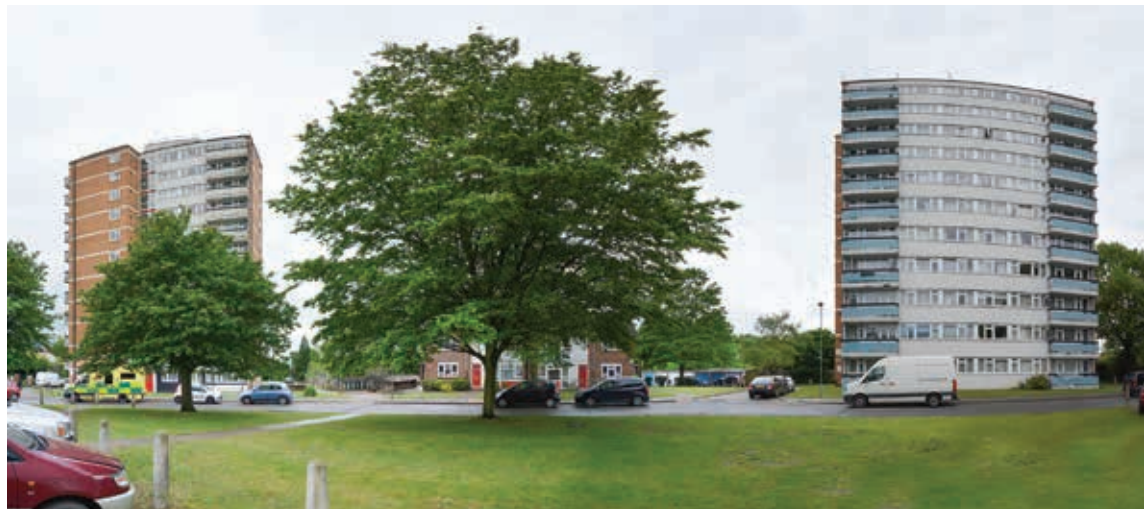
Homes and garages between the two current towers would make way for the new tower. Photo Mike Coles
