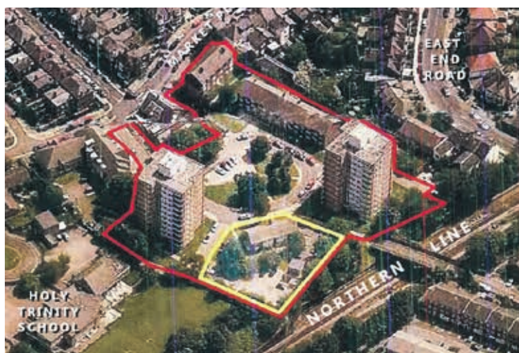
Aerial view of the proposed location of the third tower, in yellow, as displayed at the Barnet Homes consultation
