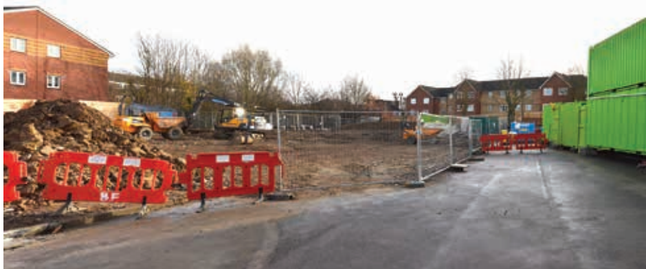
The Old Barn building site in November. Photo Mike Coles
