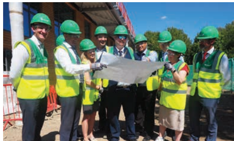
The Mayor, centre, joined ward councillors Alison Moore and Arjun Mittra at the topping out of Tarling Road Community Centre
