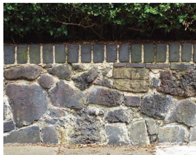
A clinker wall near Cherry Tree Wood. Photo Emily Casimir-Brown
