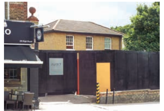
East Finchley's oldest building, Valona House
