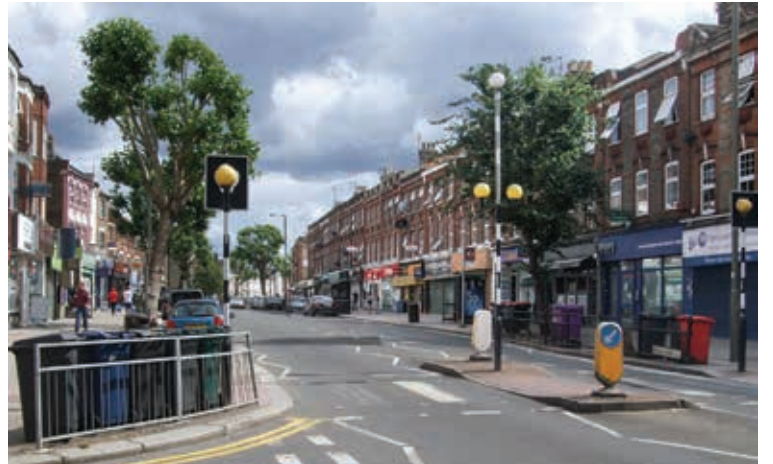
Heading south: The obscured and badly marked crossing. Photo Gill Steiner
