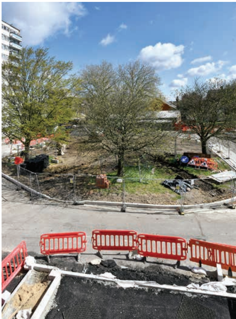
Construction work: Resurfacing and re-seeding underway in Prospect Ring.
