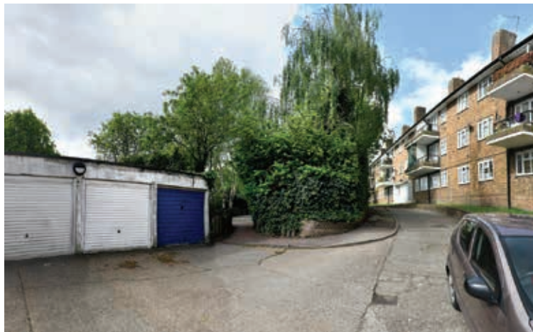
Going: A row of garages are also earmarked for demolition.
