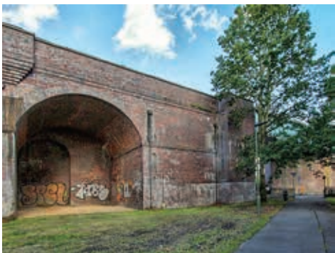
The imposing brick viaduct at Arnos Park
