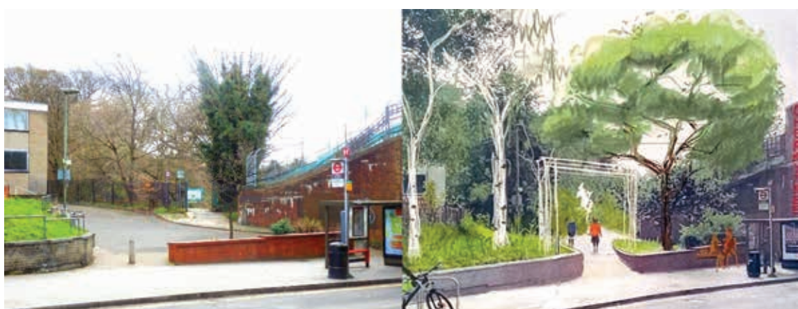
Before and after: How the wood entrance looks now, left, and an artist's impression of the new layout
