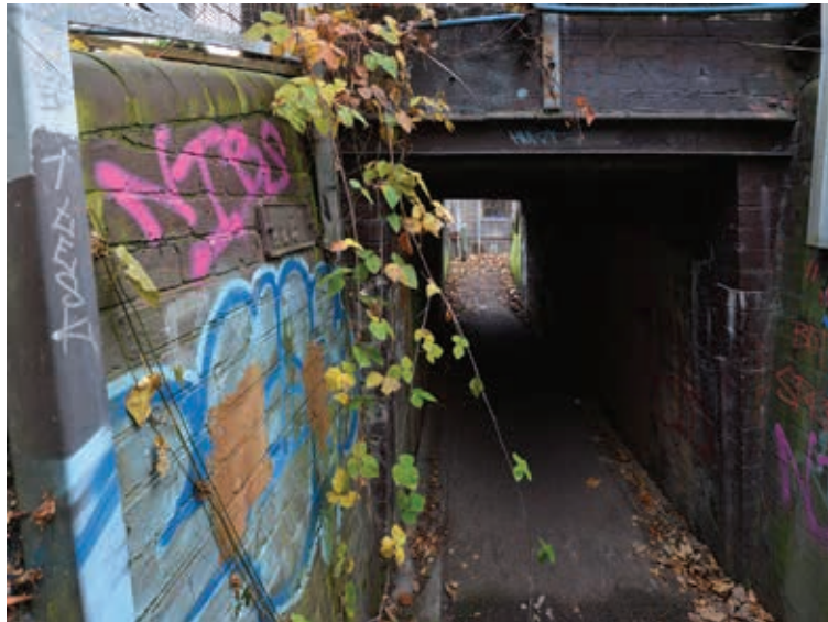
Under the tracks: The walkway passes safely under what is now the Northern line. Photo Mike Coles.
