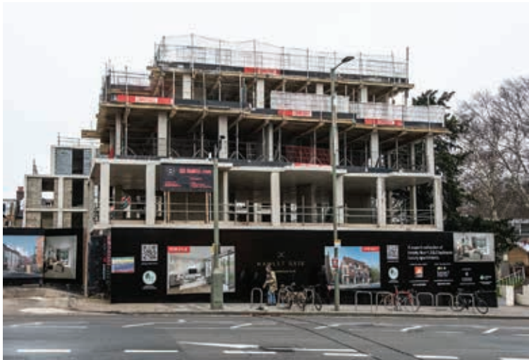
Under construction: How the High Road flats looked last month
