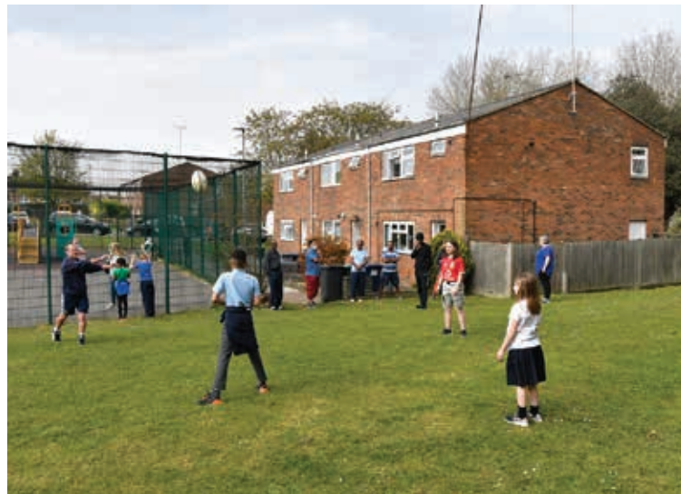
Brownswell green: Children play in front of the three homes set for demolition. Photo Mike Coles
