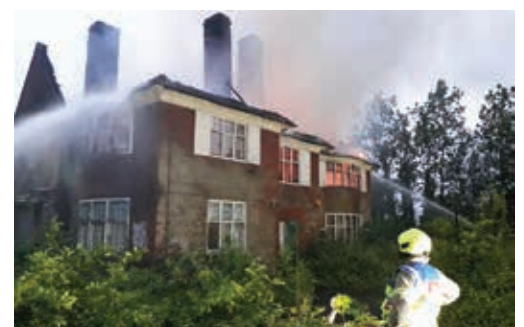
Early hours: Fire crews at the blaze on The Bishops Avenue
