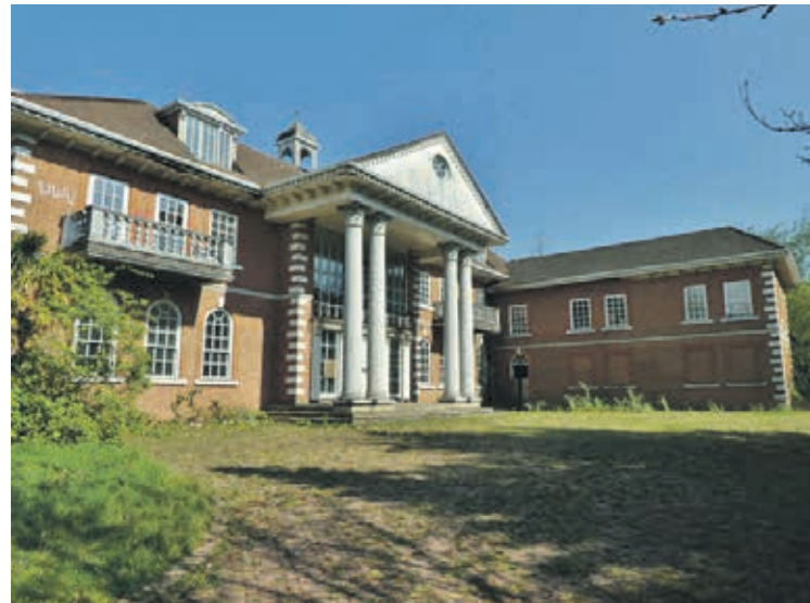
Derelict: The Towers had stood empty since it was built in the 1990s waiting for a new lease of life
