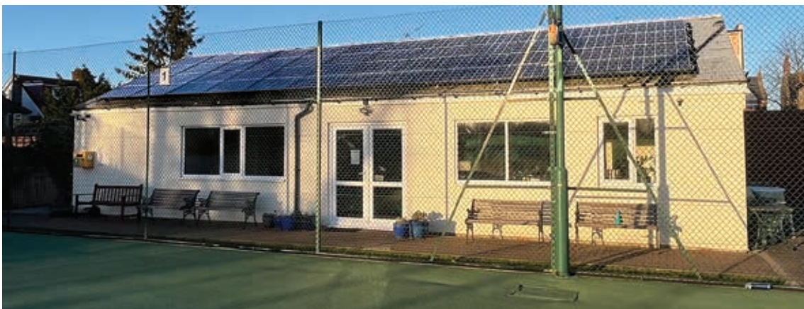
Power move: The panels on the roof of the tennis clubhouse
