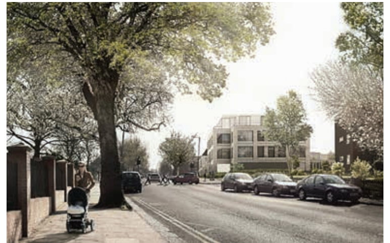
Proposals: Designs approved in 2019 would have seen the construction of 20 flats in two blocks.
