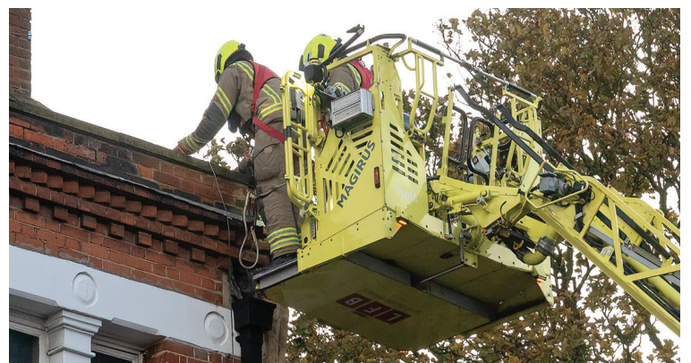
Emergency service: Firemen check the safety of the Amazing Grates rooftop following the incident there last winter. Photo Mike Coles
