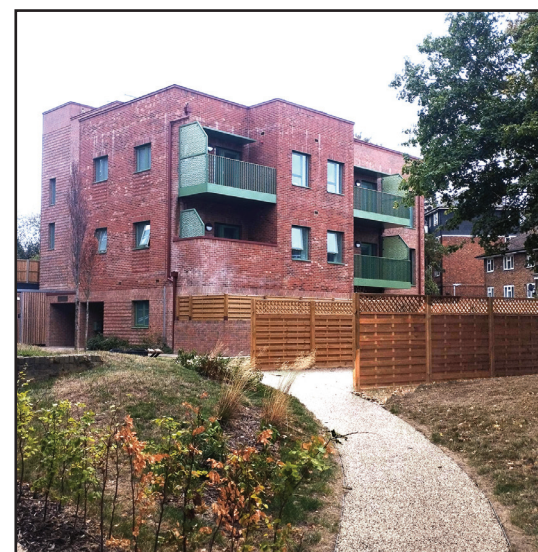
Extra homes: One of the new blocks on the Grange Estate. Photo Matteo Lanzini
